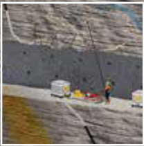
Stopping water inrush
